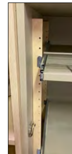
Side Mount Installation
