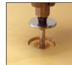
3. Countersink PowerHead screw
